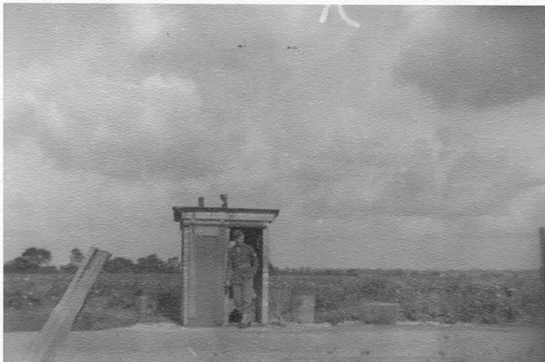
MP GATE SITE 7 36974
